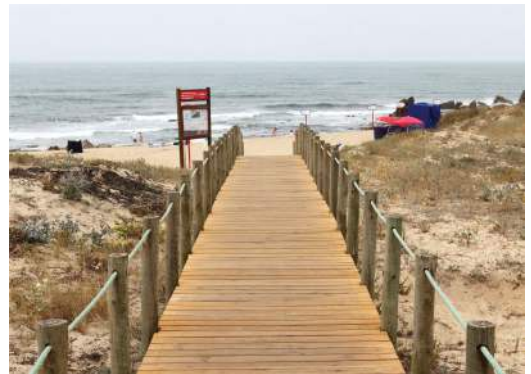
Soft engineering: area of beach replenishment north of Espinho
